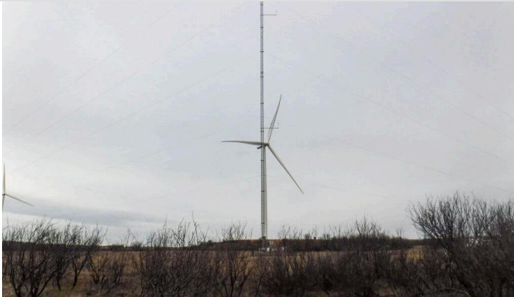
Met towers, a meteorological measurement tool used for wind siting, typically require siting permits that can take months to obtain.
